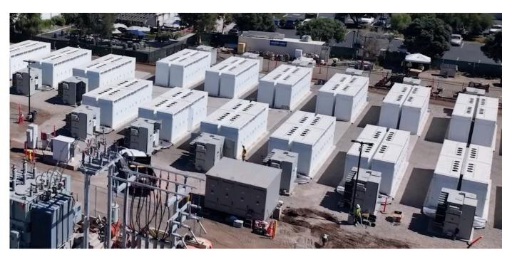
Goleta Energy Storage | Tesla | Goleta, CA 60MW/160MWh (44 Tesla Megapacks) BESS
