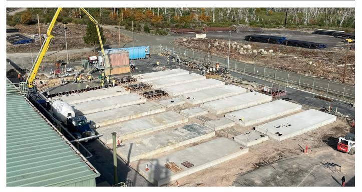
Geysers | Calpine | Middletown, CA 60MW/240MWh (re-purposed thermal plant) BESS
