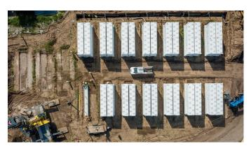
Goleta Energy Storage | Goleta, CA 60 MW BESS project 44 Tesla Megapacks BESS
