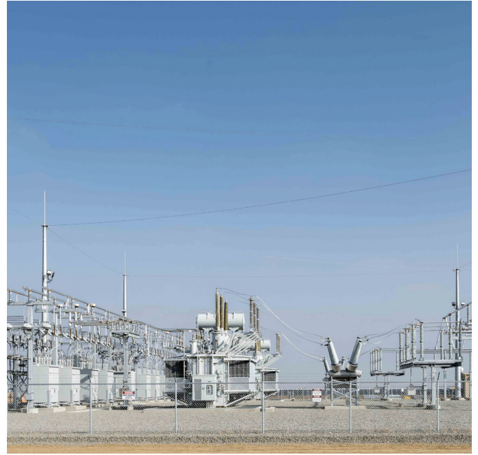
Aquamarine | SOLV Energy | Stratford, CA 250MW solar, 230kV substation Solar | Substation
