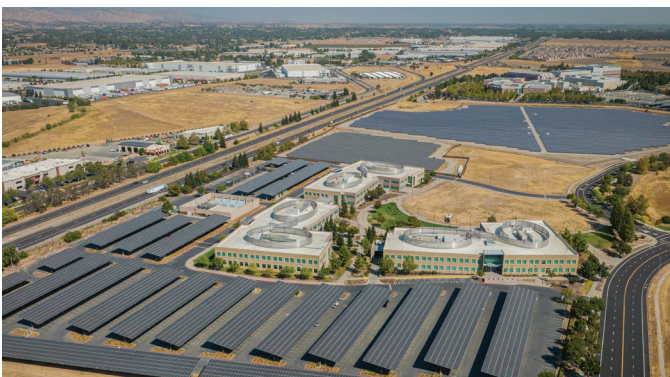
State Fund Portfolio | Vacaville, CA 10.6 MW distributed generation across 4 sites: Vacaville, Pleasanton, Redding, Sacramento Solar | EV Charging | BESS
