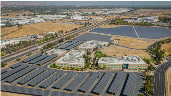
State Fund Portfolio | Vacaville, CA 10.6 MW distributed generation across 4 sites: Vacaville, Pleasanton, Redding, Sacramento Solar | EV Charging | BESS
