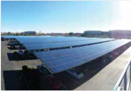
Solar City/Intel Folsom 6MW solar and 1MW/2MWh battery Renewable energy / solar Electrical construction including battery plant, solar and parking canopies.
