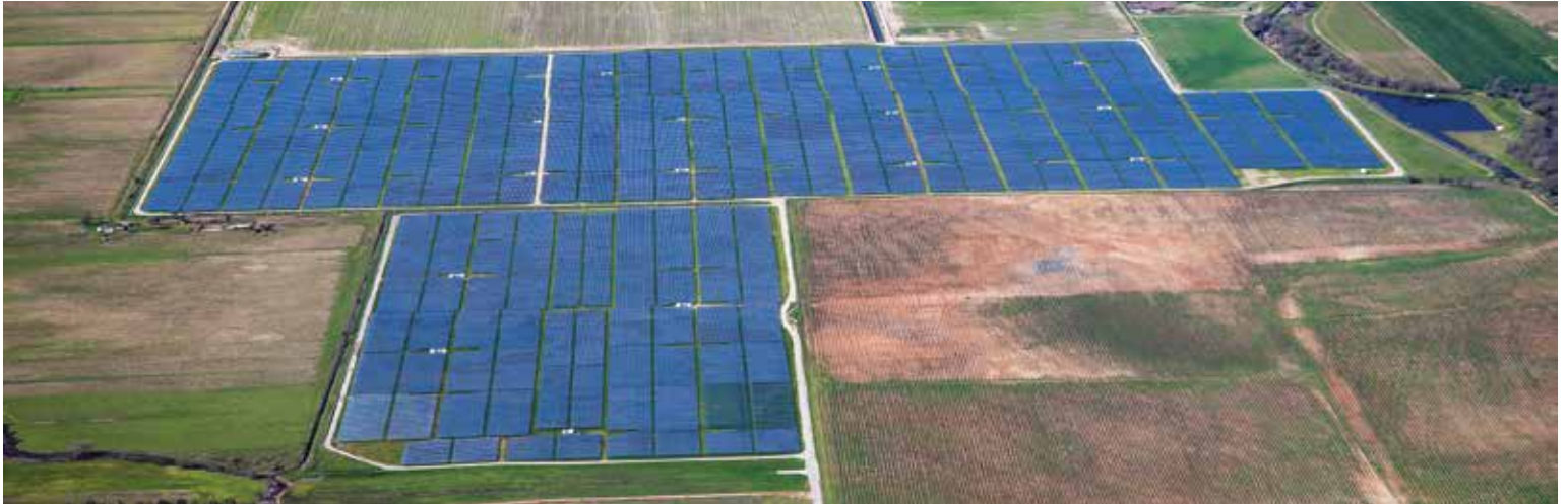
McKenzie Power Plant | Galt, CA 2013 | 30 MW
